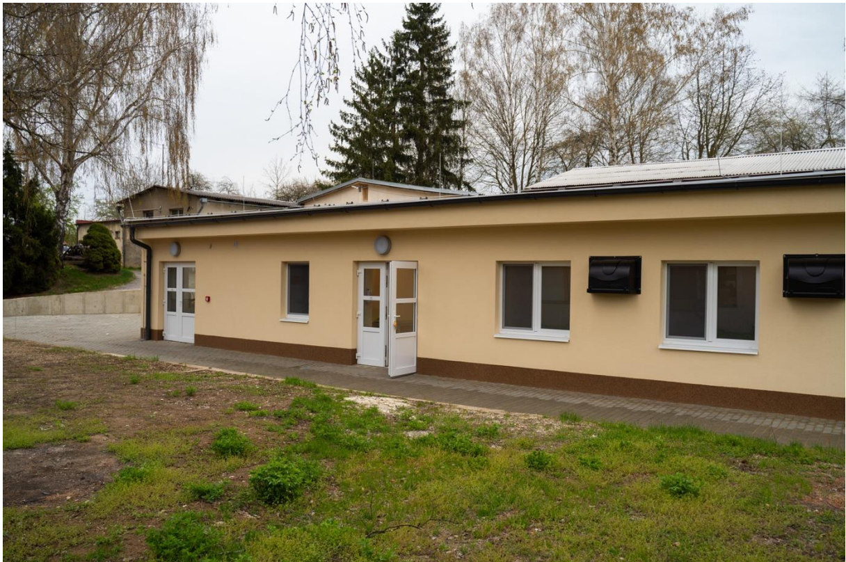
Renovated poultry farm building at the IMG detached site in Koleč. (Author: M. Jakubec, IMG)
